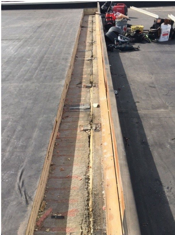
Left: Workers cut this section of the core library roof out so they could cut the welded plate (photo on the right) between the roof panel Ts, freeing up the east-west panels to be welded directly to the underlying steel beam.
