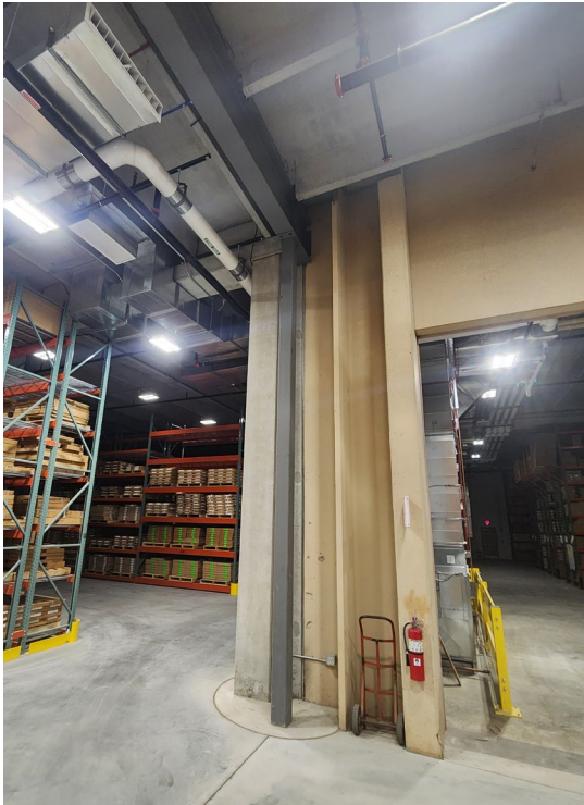
Left: The steel post sits outside of the southwest corner of the original core library, the steel beam above it runs north-south. Above: The area where the roof panels were moving and cracking on the ends is circled in red. The steel beams (blue lines) to the south of the old warehouse run north and south while the concrete beams throughout both the rest of the expansion and the old warehouse are oriented east - west.
