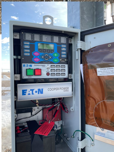
Northern Plains Electric Cooperative completed their IIJA grant project in April 2025, the installation of several SCADA ready reclosers. The state of the art recloser control panel and a completed substation are pictured above.
