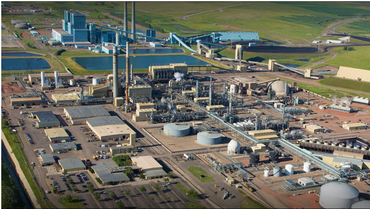
The Synfuels Plant will be reconfigured to utilize natural gas to produce synthesis gas (syngas) and then modify the existing product slate to produce hydrogen as a low carbon intensity fuel for internal use, electric power production, blending into existing natural gas pipelines, existing and expanded ammonia production and other transportation and industrial applications.
