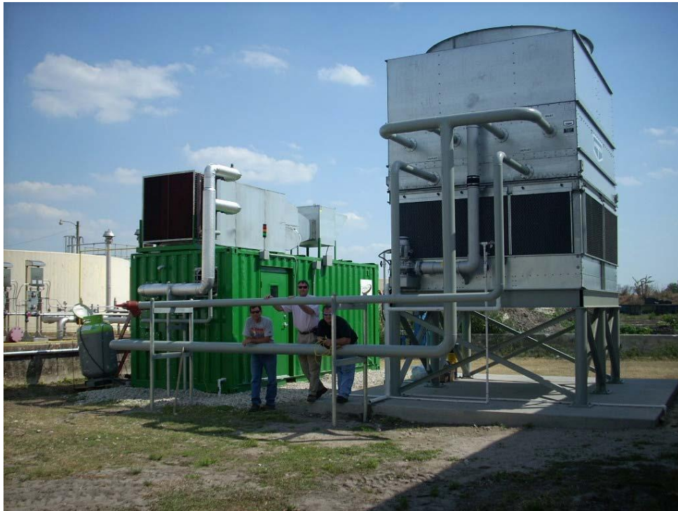
Figure 4 Application of Calnetix WHG100 waste heat recovery generator
