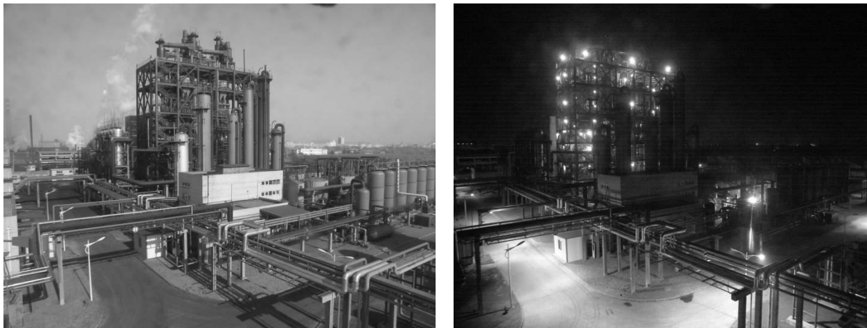
Figure 2.4.4. U-GAS ® Hai Hua Gasification Facility in China Built by SES (GTI, 2009)
