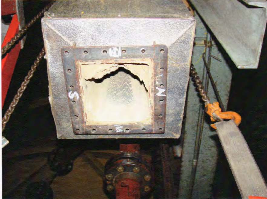
Figure 4. Inlet to the catalyst section of the SCR reactor view looking upstream; Coyote Station at the 2-month test interval.
