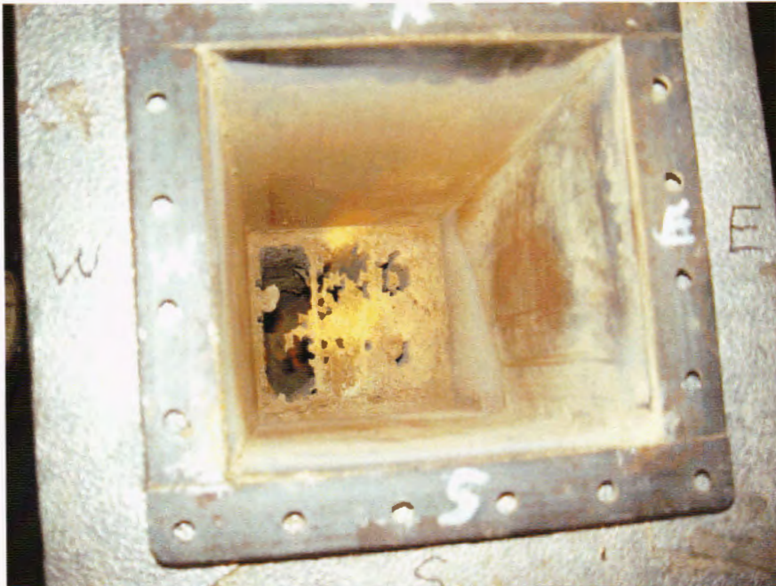
Figure 7. Inlet of the catalyst section of the SCR reactor after catalysts have been removed; view looking downstream; Coyote Station at the 2-month test interval.
