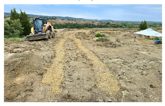
Survey paleontologists removed the wet clay with shovels and built a two-track using the dry rock the grader had churned up. The skid-steer loader, from the construction company working on the TR Presidential Library, is stuck along the edge of the entrance into the dig site.
