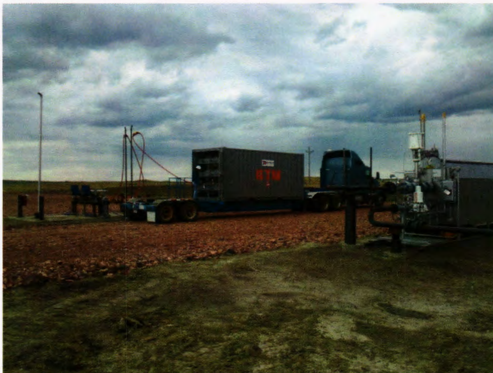
Unloading First Tube Container
