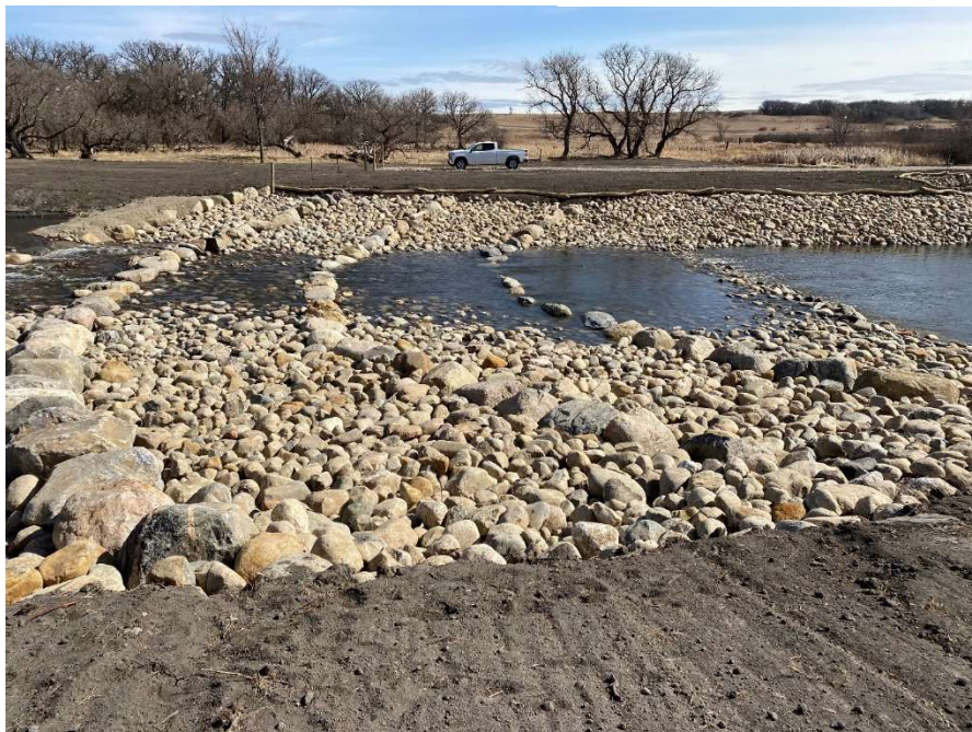
Figure 2 (04-08-2021) – Riprap High Point Downstream of Final Riffle
