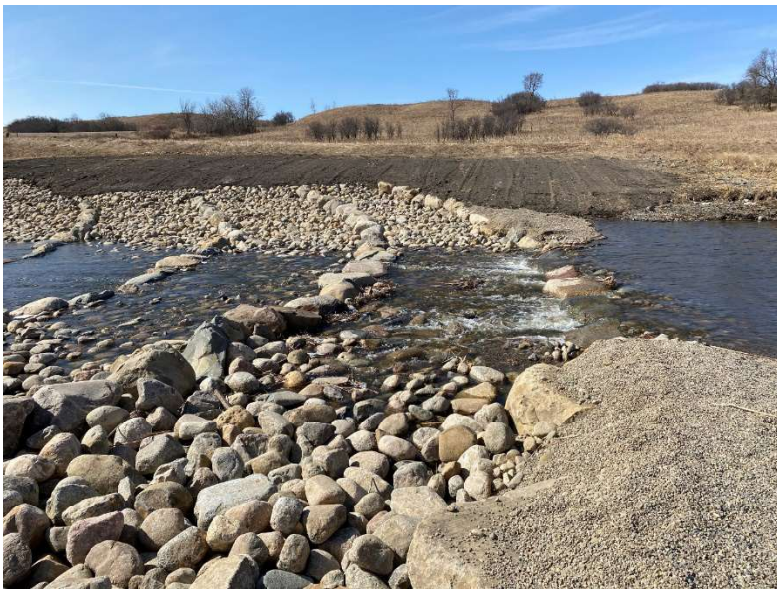
Figure 4 (08-04-2021) – Erosion Control on Right Bank U/S of the Riffle Structure
