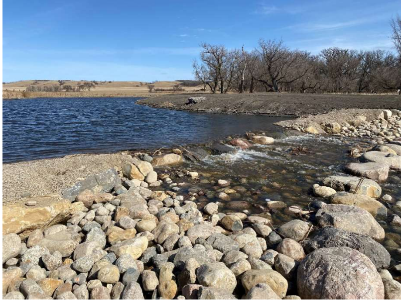
Figure 3 (04-08-2021) – Erosion Control on Left Bank U/S of the Riffle Structure
