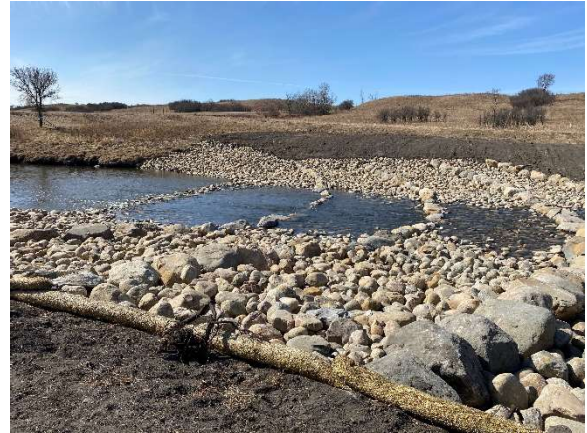
Figure 1 (04-08-2021) - Rock Riffle structure
