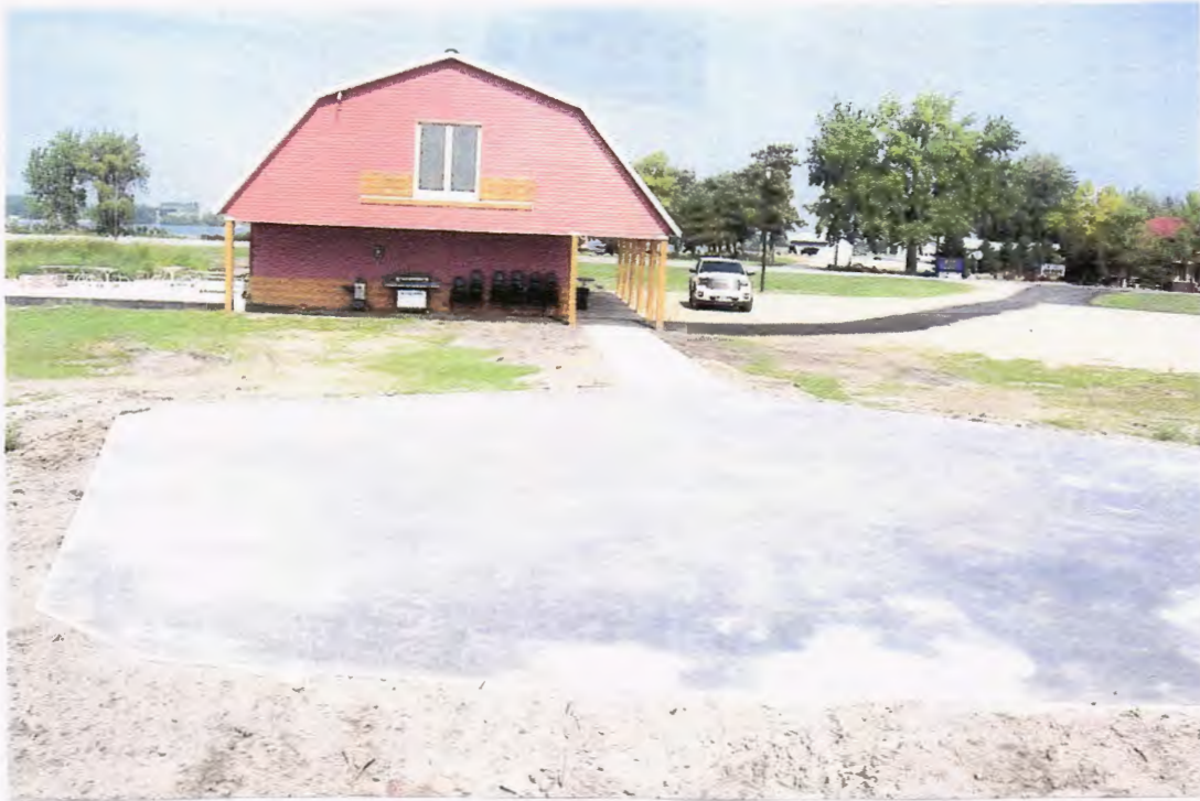
CONCRETE SLAB FOR OUTDOOR CLASSROOM/AMPHITHEATER SOUTH OF INDOOR CLASSROOM/COMMUNITY BUILDING
