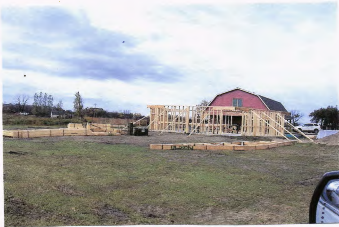
CONSTRUCTION OF WALLS ON PENTAGON SHAPED BUILDING FROM SOUTH EXPOSURE.
