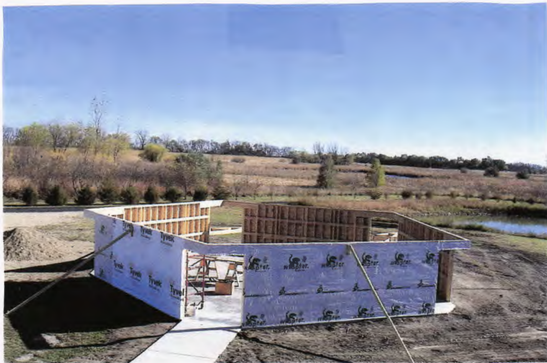
WALLS ERECTED, SHEETED AND WRAPPED AWAITING SIDING AND RAFTERS
