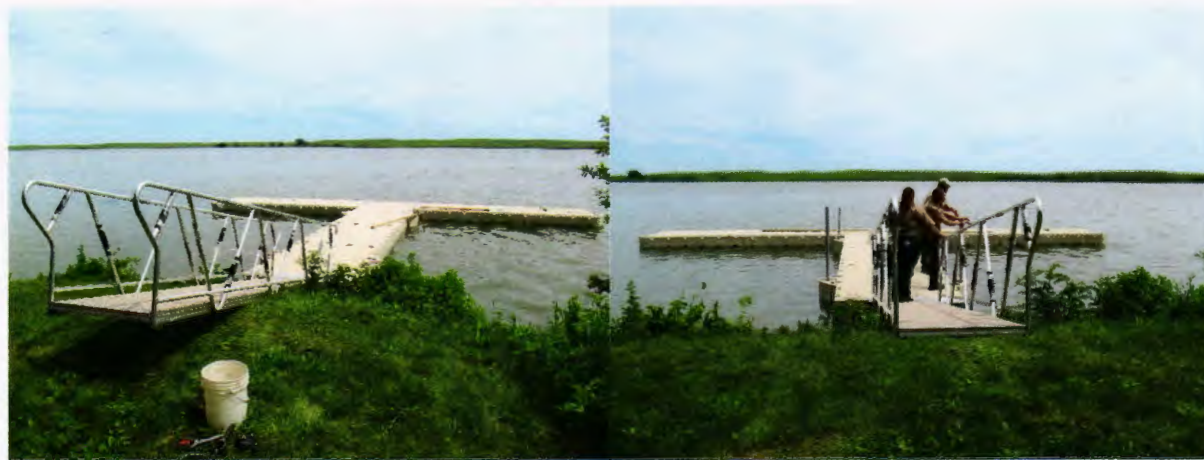
Photos 21 - 22: Gangway installation complete.
