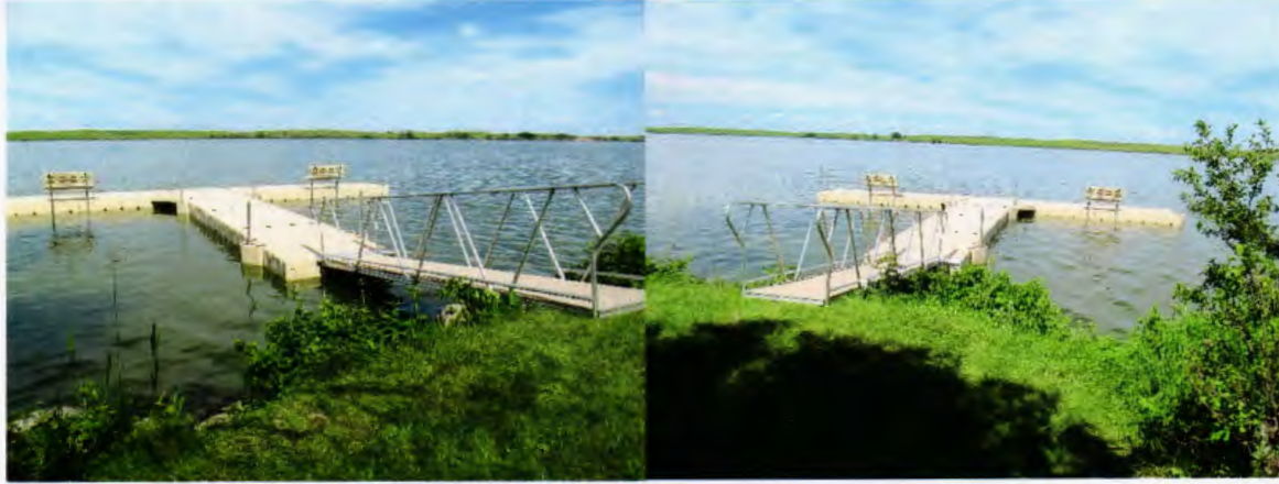
Photos 29 – 30: Completed dock in the Memorial Picnic area.
