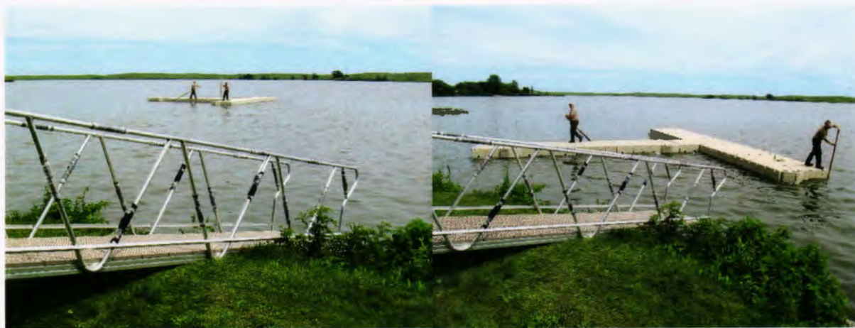
Photos 17 – 20: The long ride to the install site.
