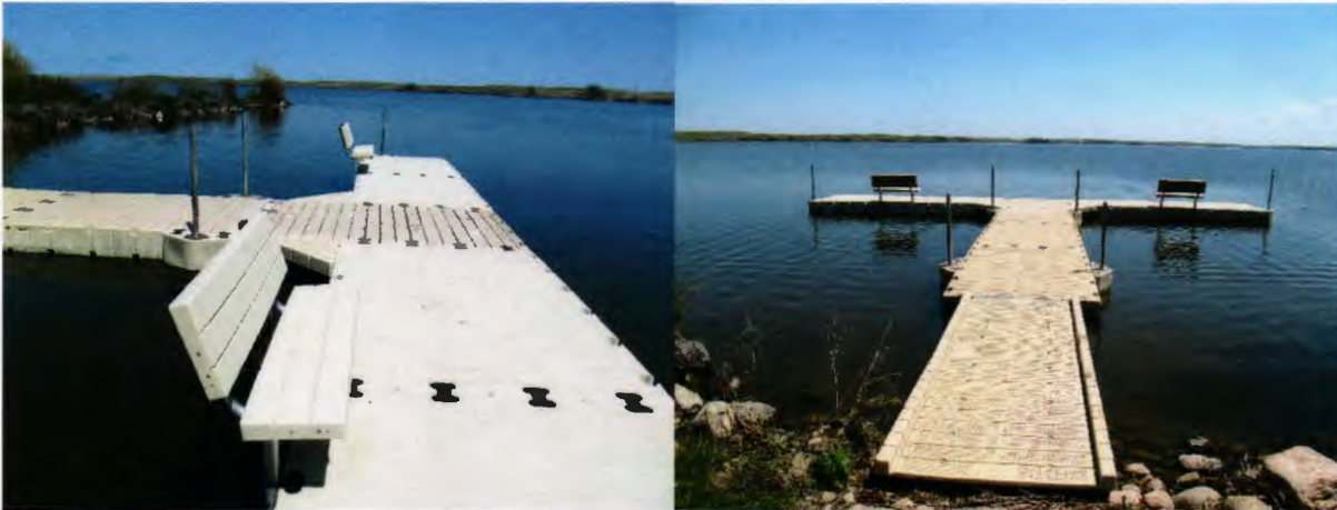
Photos 9 & 10: Completed fishing dock expansion.
