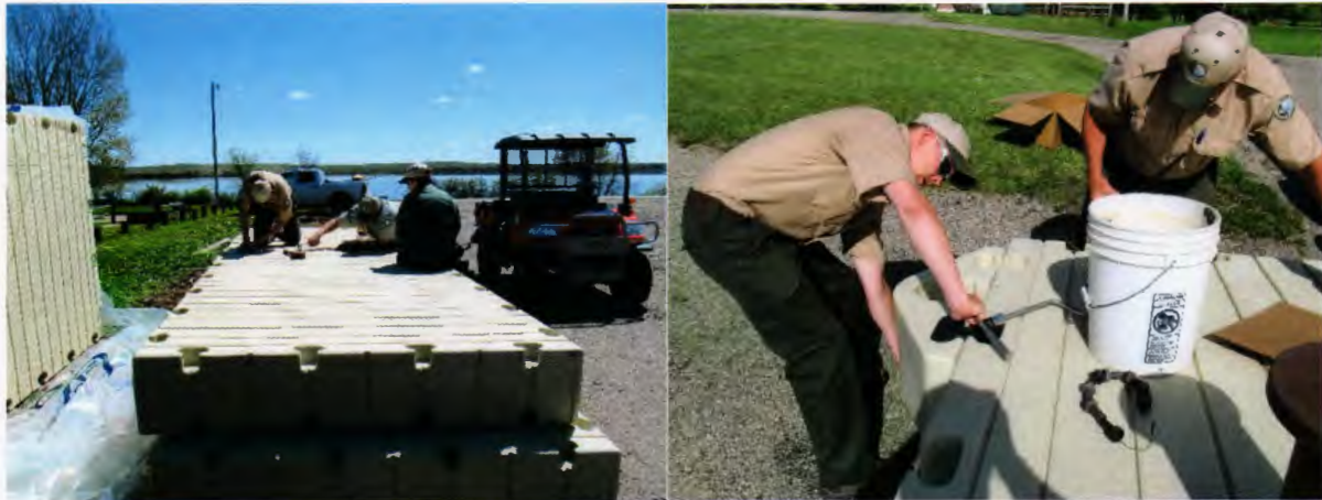
Photos 3 & 4: Preassembly of the dock sections.
