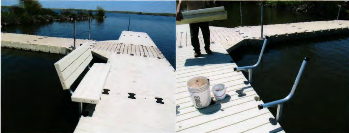
Photos 7 & 8: Installation of the corner gussets and benches.
