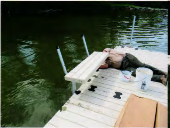
Photos 27 – 28: Bench and gusset installation.
