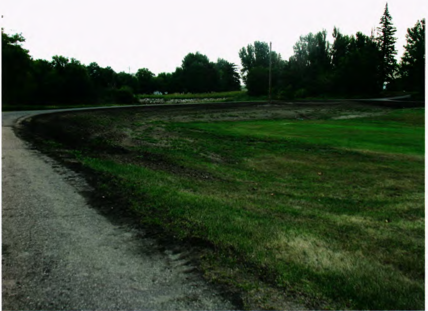
Finished Road Raise
