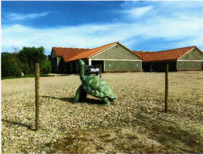
Water well loction is under turtle in parking lot.
