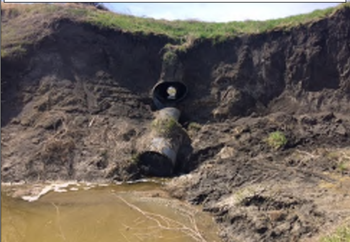
Drain 22 Outlet: Recent bank erosion
