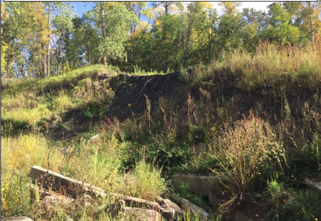
Drain 22B Outlet: Recent bank erosion
