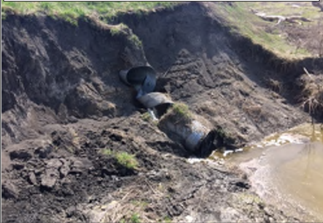
Drain 22 Outlet: Recent bank erosion
