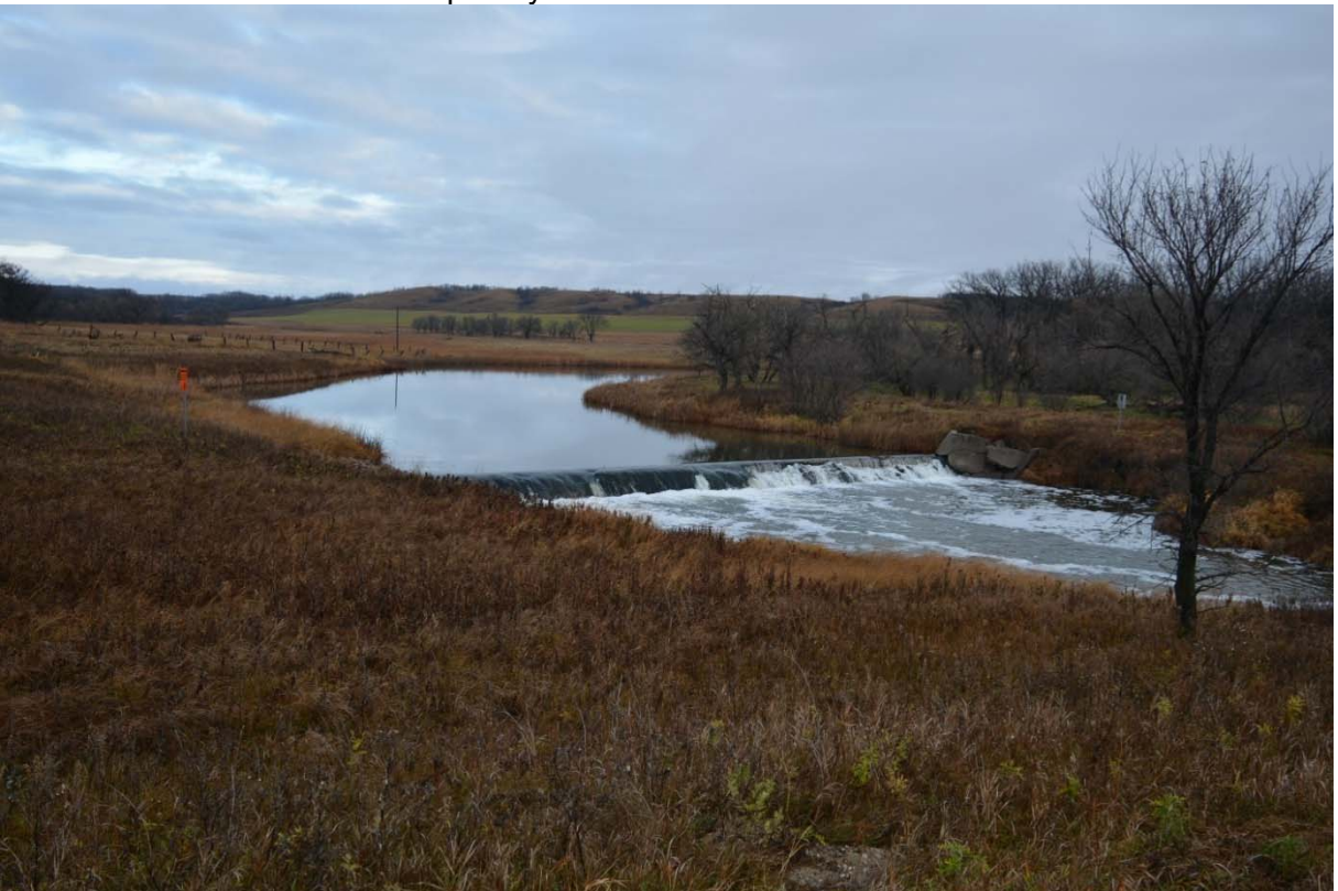
Photo 4: Bouret Dam 01-11-2016 Side view of spillway
