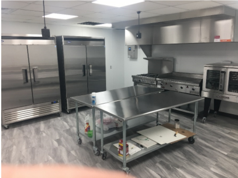
New Scout Facility Commercial Kitchen
