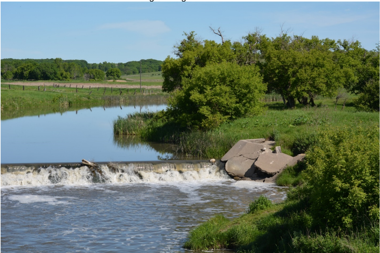
Photo 2: Bouret Dam 06-07-2016 Eroded river left abutment
