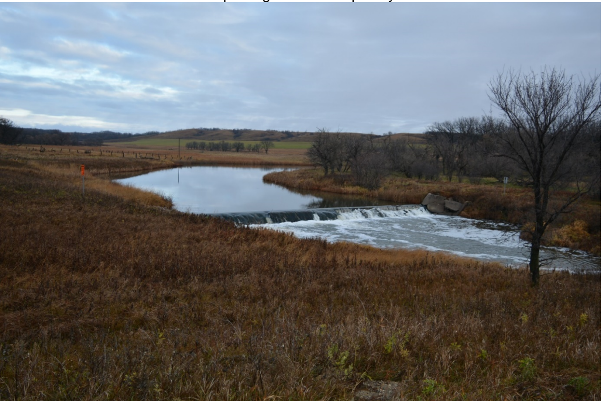
Photo 4: Bouret Dam 01-11-2016 Side view of fish passage barrier at the spillway
