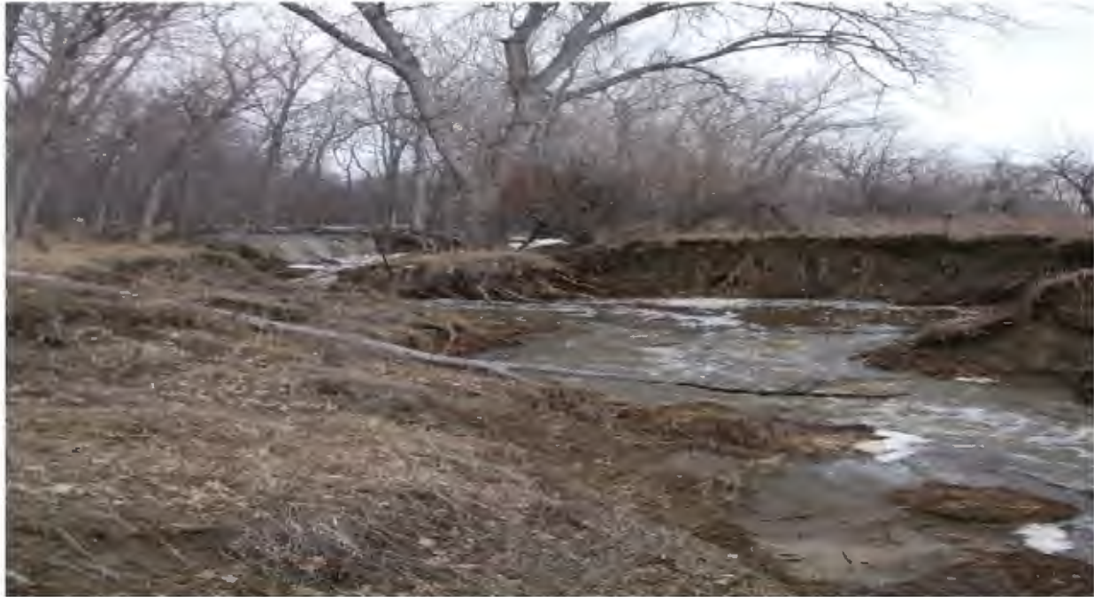
Example Flood Damages In Fort Mandan Park
