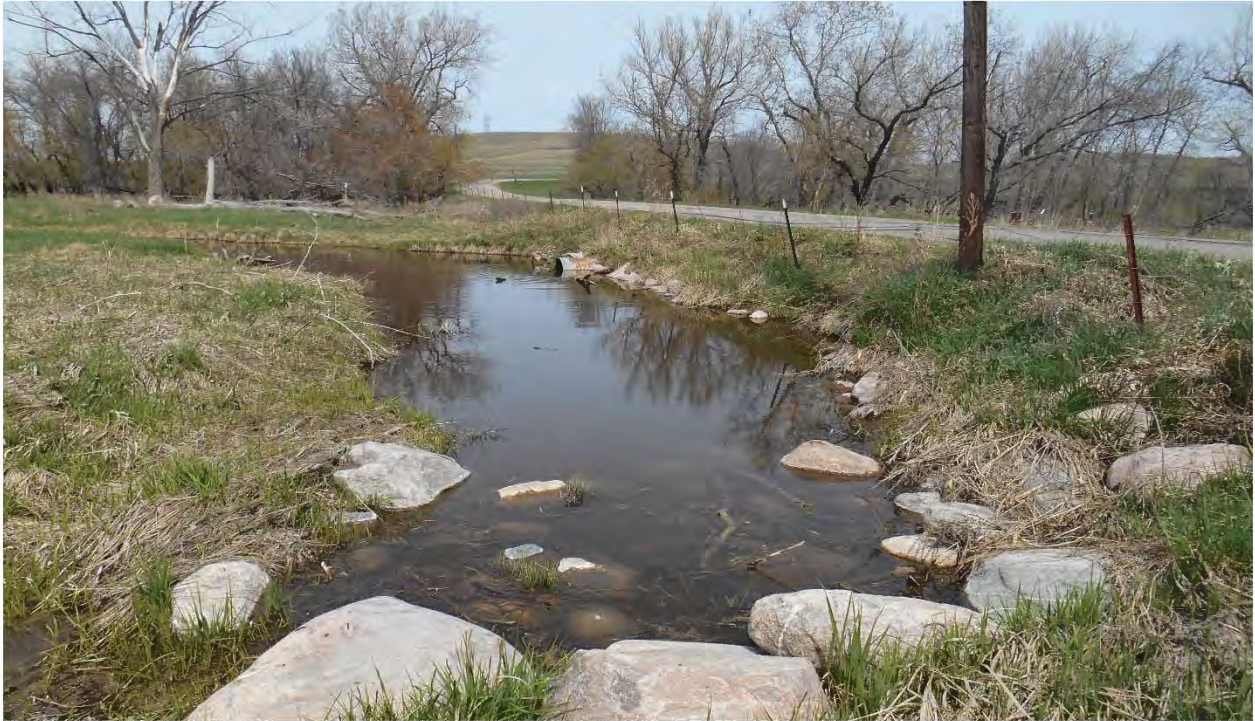
Fort Mandan Access Road at Buffalo Creek
