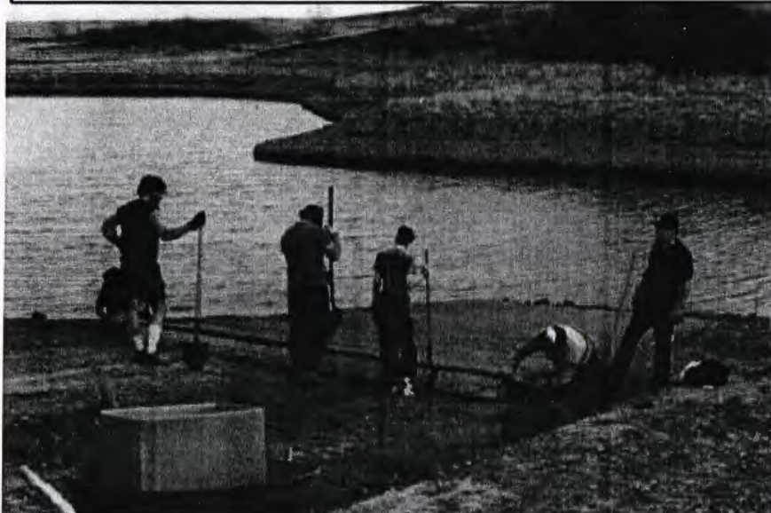
Photo #3 = Slab "A" has been poured and is being finished. Again, note the rebar left sticking out the top form which will be bent upward when Slab "A" is pushed out into the water.
