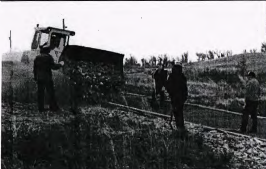
Photo #7 = Slab "B" has been poured in place and will be allowed to properly cure. Rock is being placed along both sides of the ramp to prevent any erosion and undermining from occurring. Rock utilized as rip-rap should not exceed 2' in diameter and once placed should not be higher than the surface of the ramp.
