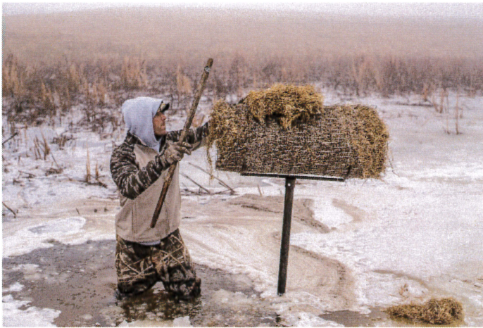
Figure 1. A contractor maintains a Hen House near Woodworth, North Dakota. Fresh flax straw ensures the structure is ready for nesting hens.
