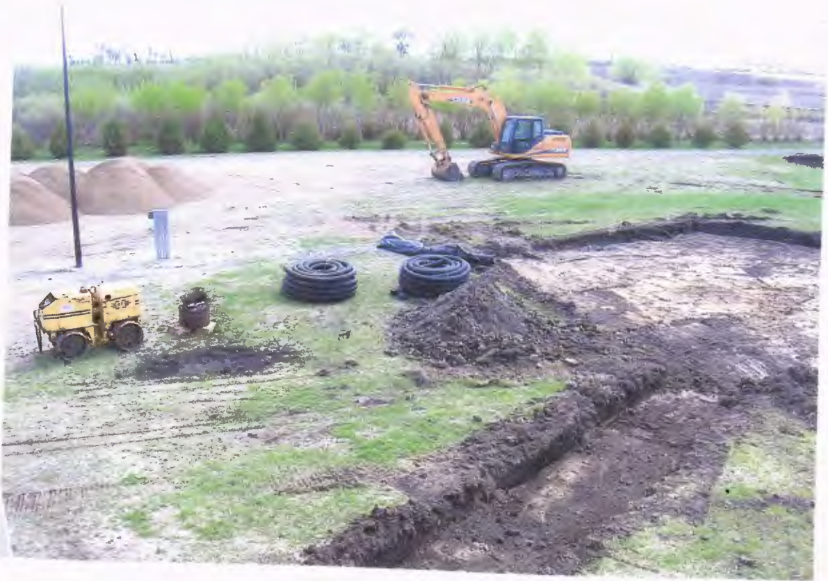
GEO TEXTILE FABRIC, PIPE, GRAVEL AND EXCAVATION PREPARING FOR BASE CONCRETE
