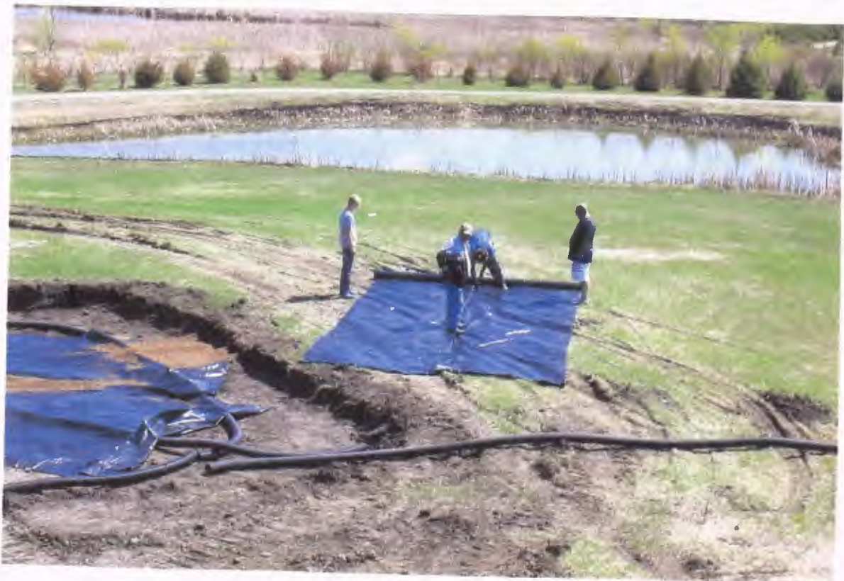
INSTALLATION OF GEO TEXTILE FABRIC AND PIPING
