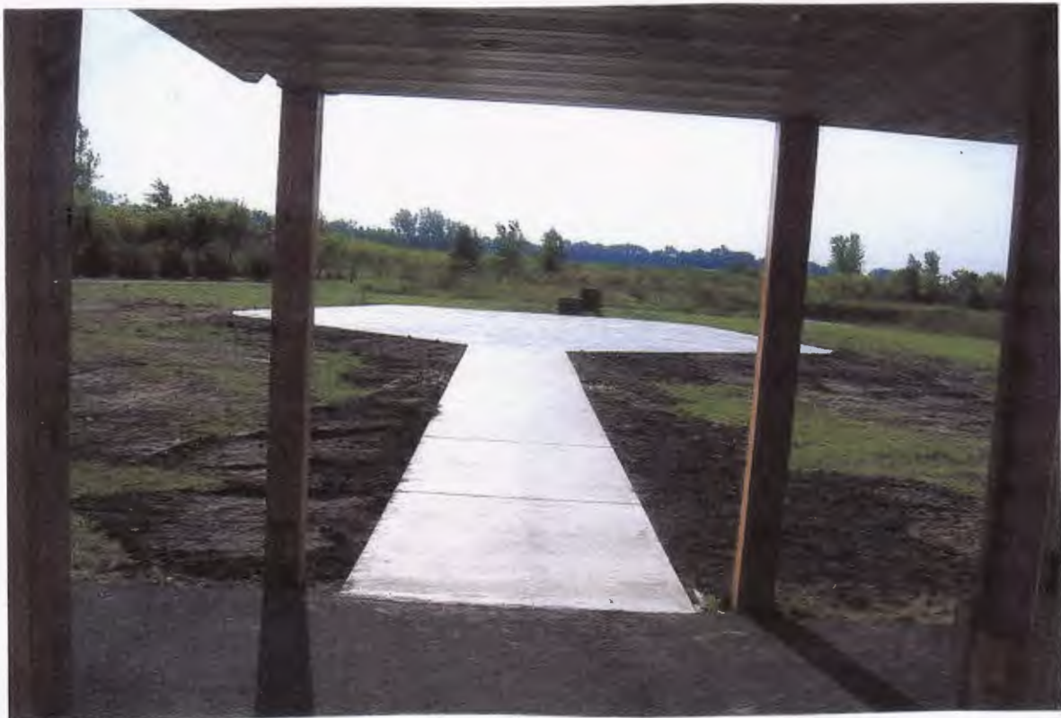
COMPLETED HANDICAPPED ACCESSIBLE CONCRETE BASE FOR OUTDOOR CLASSROOM/AMPHITHEATER
