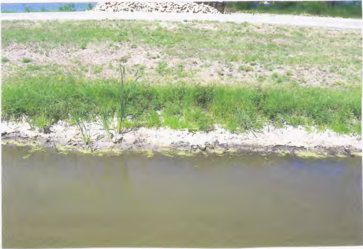
1. SHORELINE-NORTH SIDE OF CHANNEL PRIOR TO INSTALLING ROCK RIPRAP.
