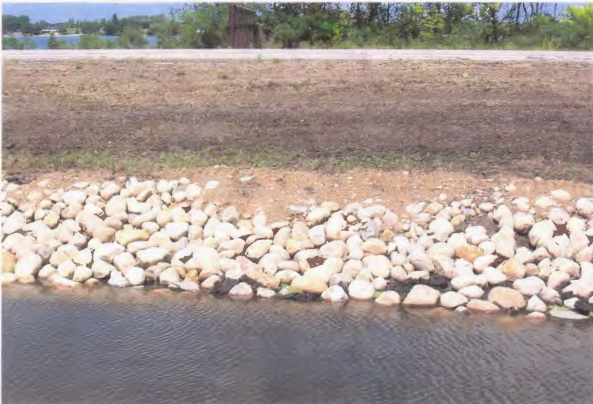
4. SHORELINE SHOWING GRAVEL BASE FOR ROCK RIPRAP.
