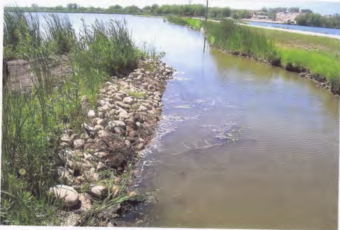
2. SHORELINE-SOUTH SIDE OF CHANNEL WITH ROCK RIPRAP.
