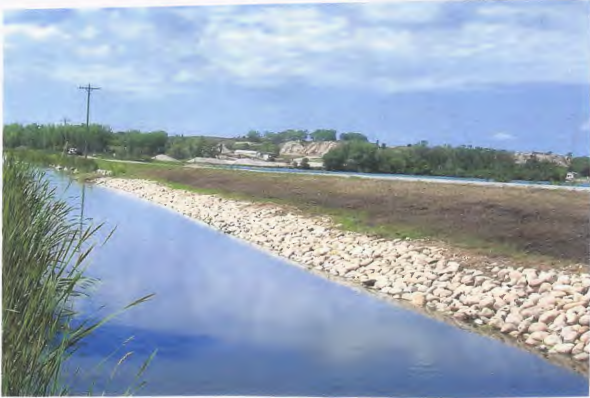
3. SHORELINE-NORTH SIDE OF CHANNEL WITH COMPLETE RIPRAP.
