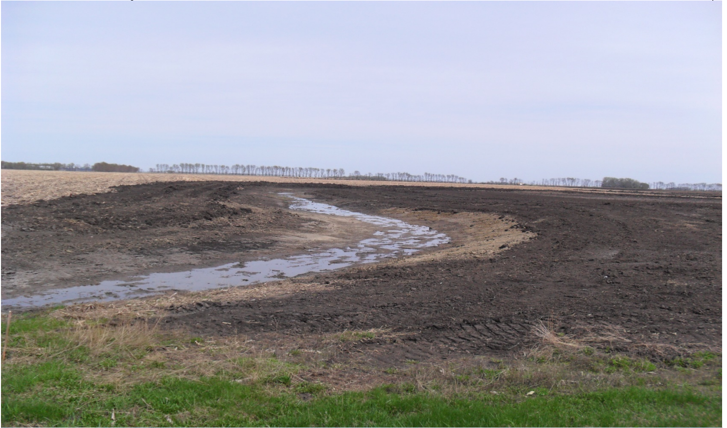
Photo of work completed and seeded 5/2018–
