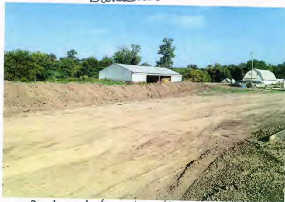
Dirtwork / water line install
