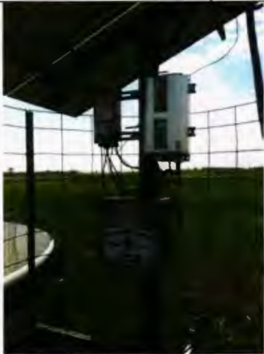
All controls protected by panels
