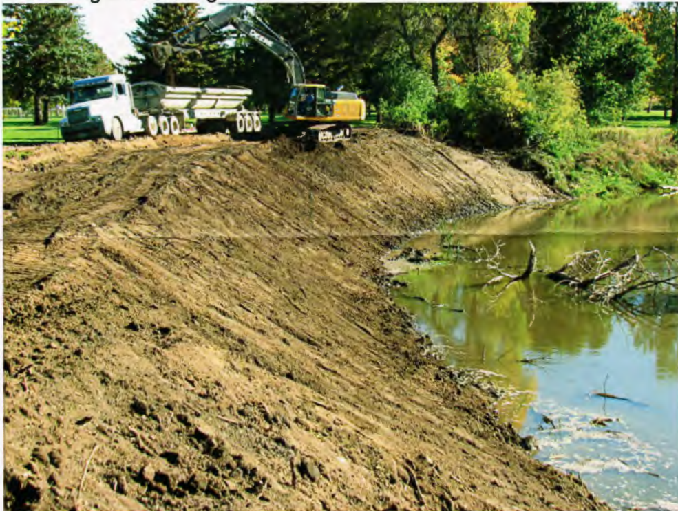
Excavating and Grading
