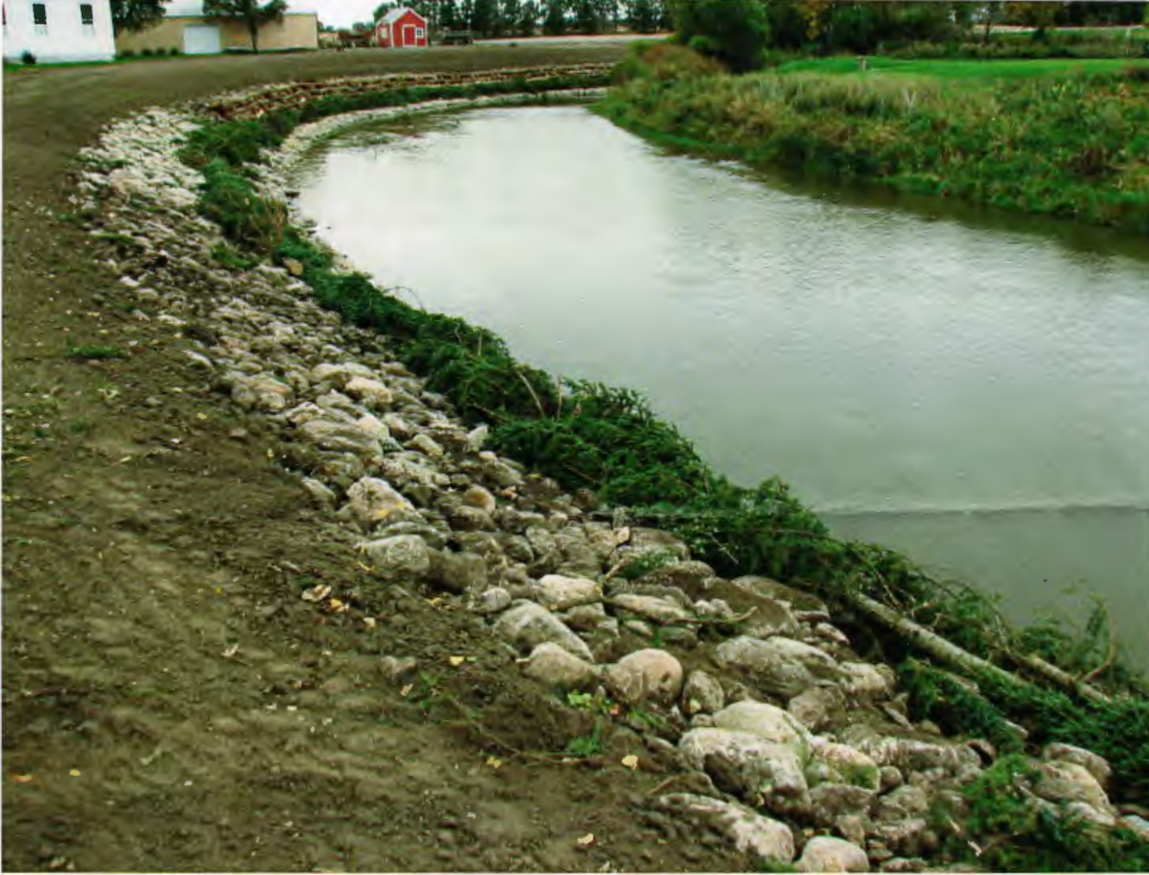
Conifer Revetment placement
