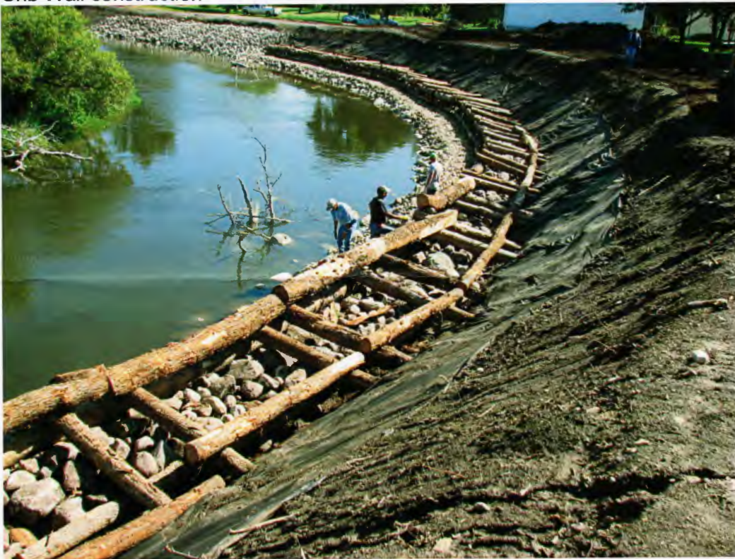
Crib Wall construction
