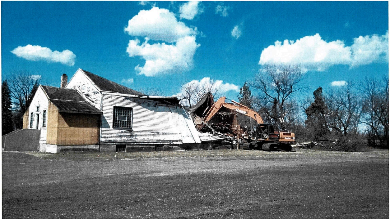
Demolition began on morning of April 13, 2015.
