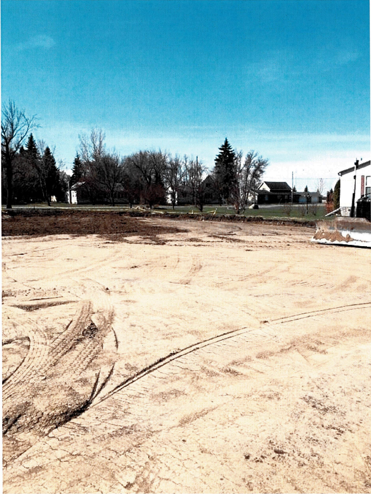
Clay was brought in on Wednesday, April 29 and pad construction began.
