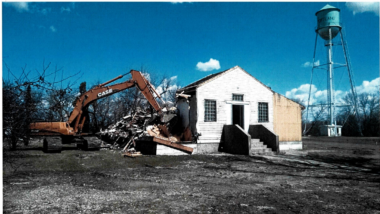
Within hours the building was nearly demolished.
