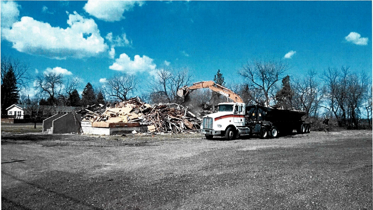
Contractors were removing debris from the site immediately following demolition.
