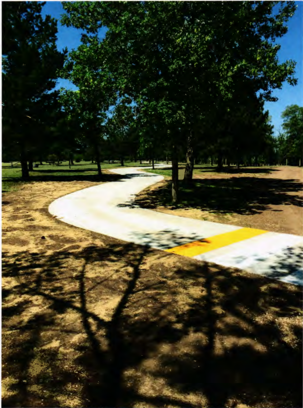
Figure 3 - New Concrete Trail Through Campsite Area
