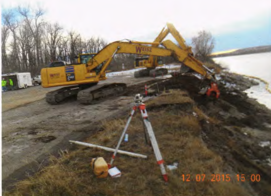
Compacting backfill
