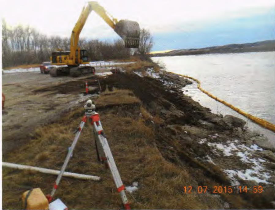
Backfilling
