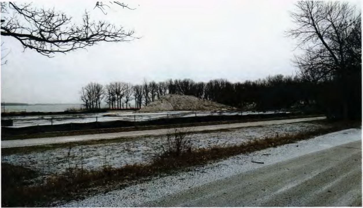
Stockpile of materials in the baseball field
