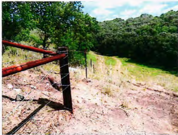
20,668 foot fencing project
