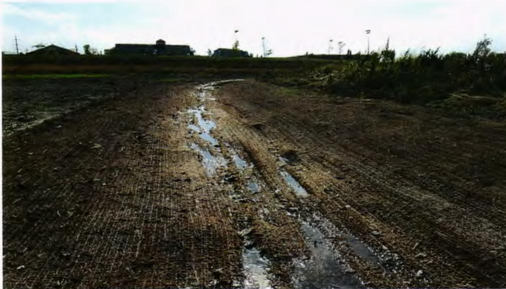
Interim erosion control for disturbed areas. Existing grade on right is more of a water barrier than originally expected. Force of water movement in new channel is stronger than expected, October 2015.
