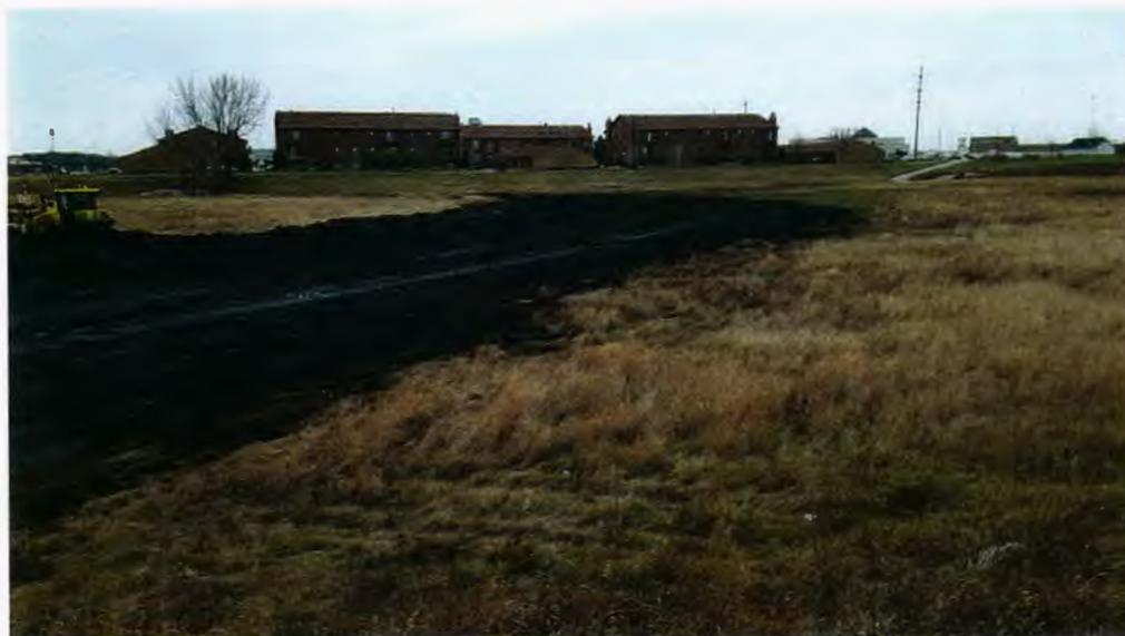
Finished grading as contractor ends up having to widen the new channel in order to create better water flow for less erosion and more natural conditions for easier vegetation establishment, November 2015.
