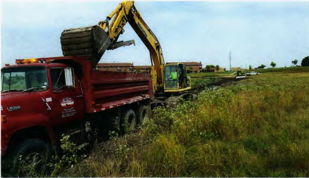
Concrete channel being removed. The contractor started at the north end and had to carefully consider sequencing in order to minimize disturbance, September 2015
