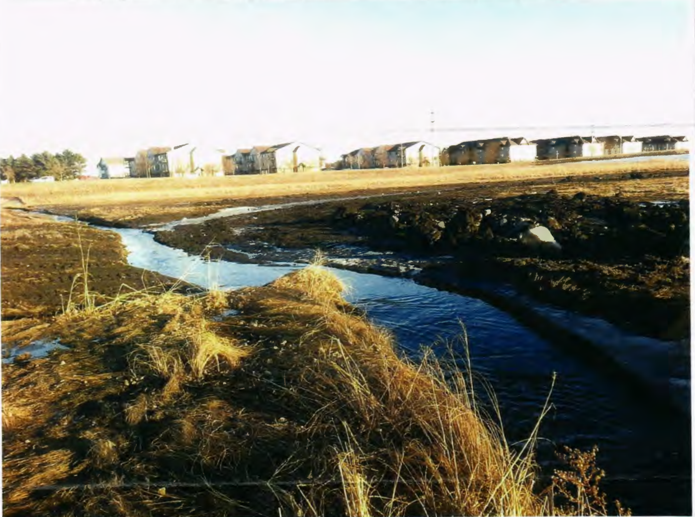
Channel, concrete removed, March 2016
