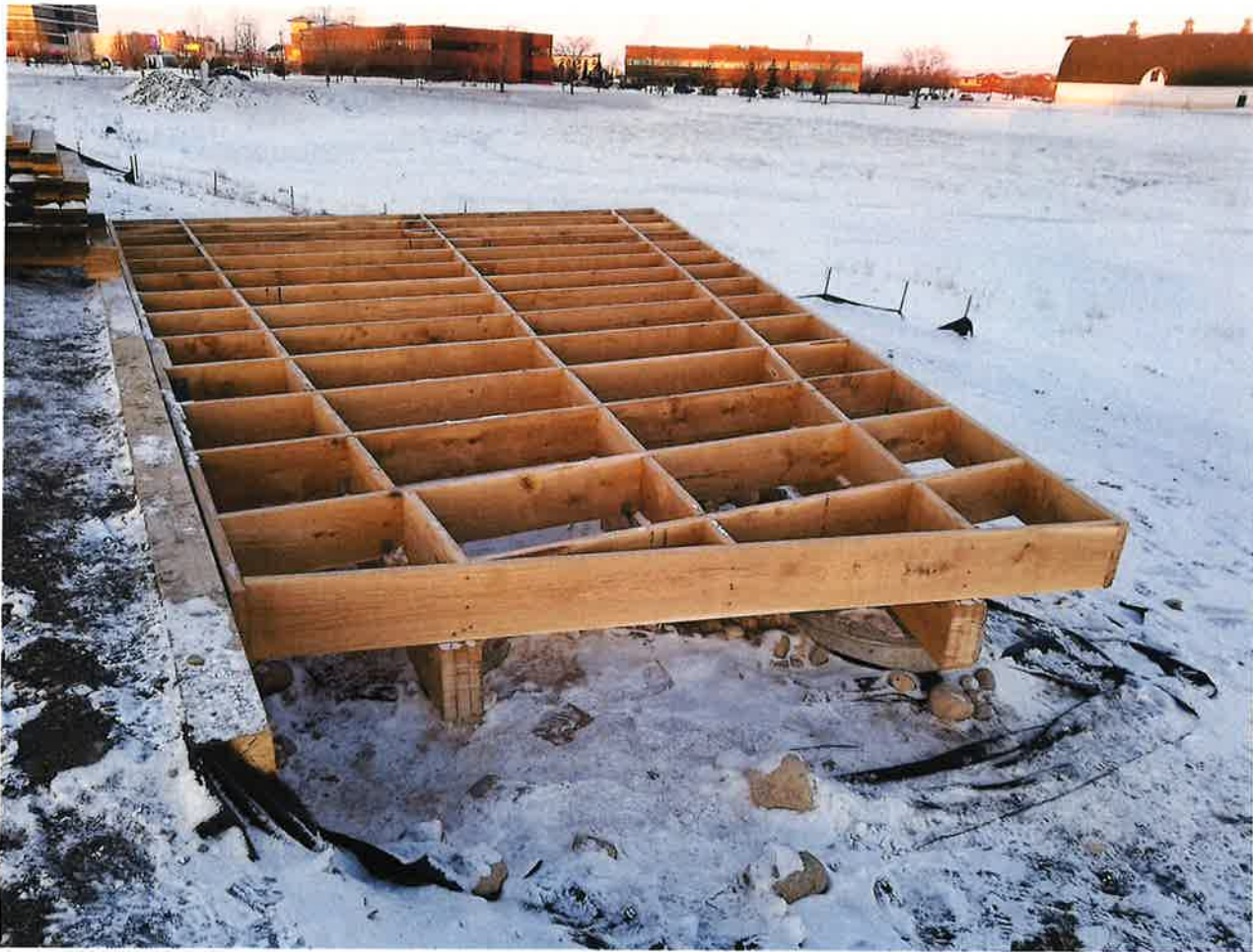
Construction of Overlook - February 2018
