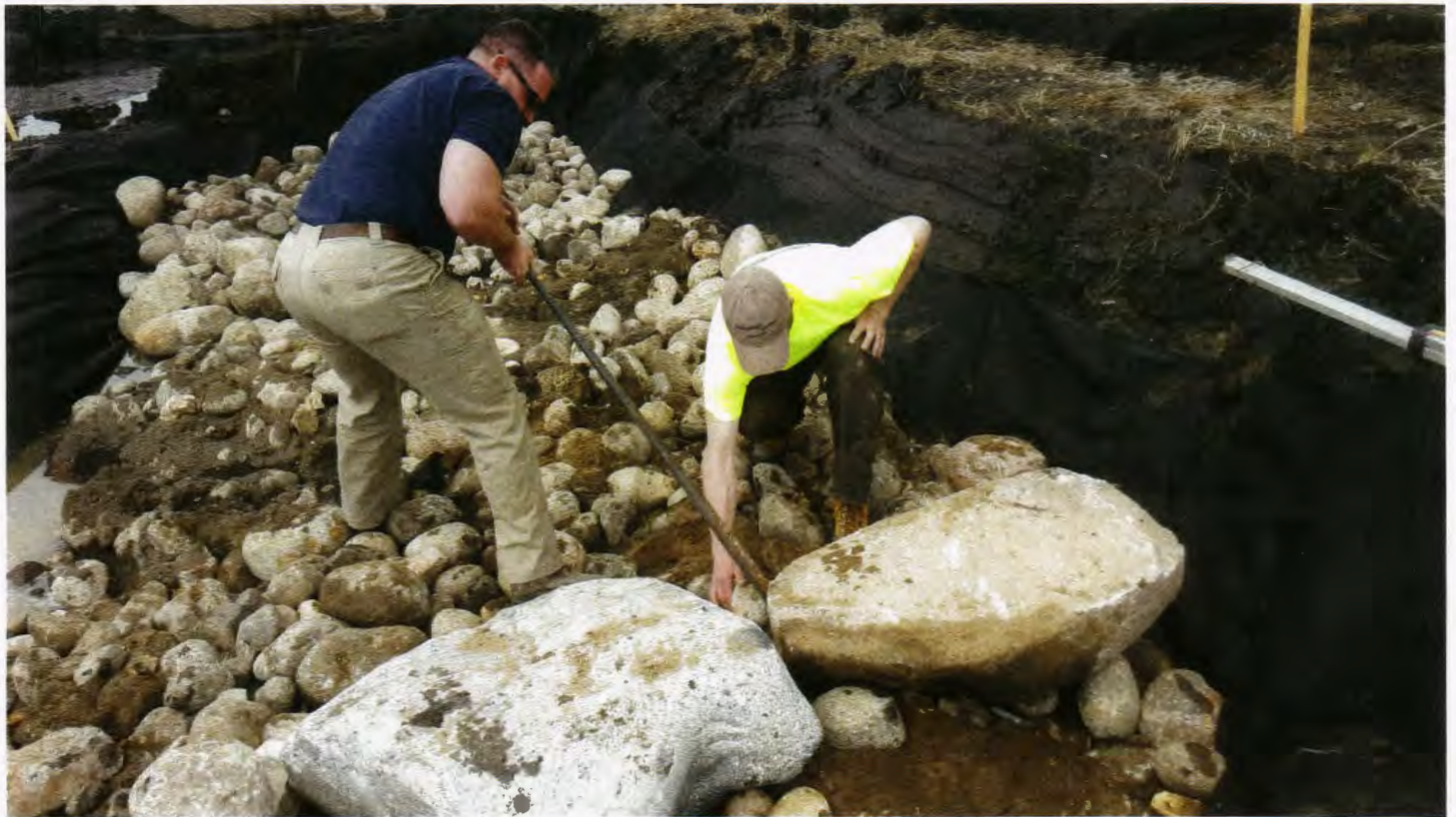
Construction of Rock Vane (April 2016)
