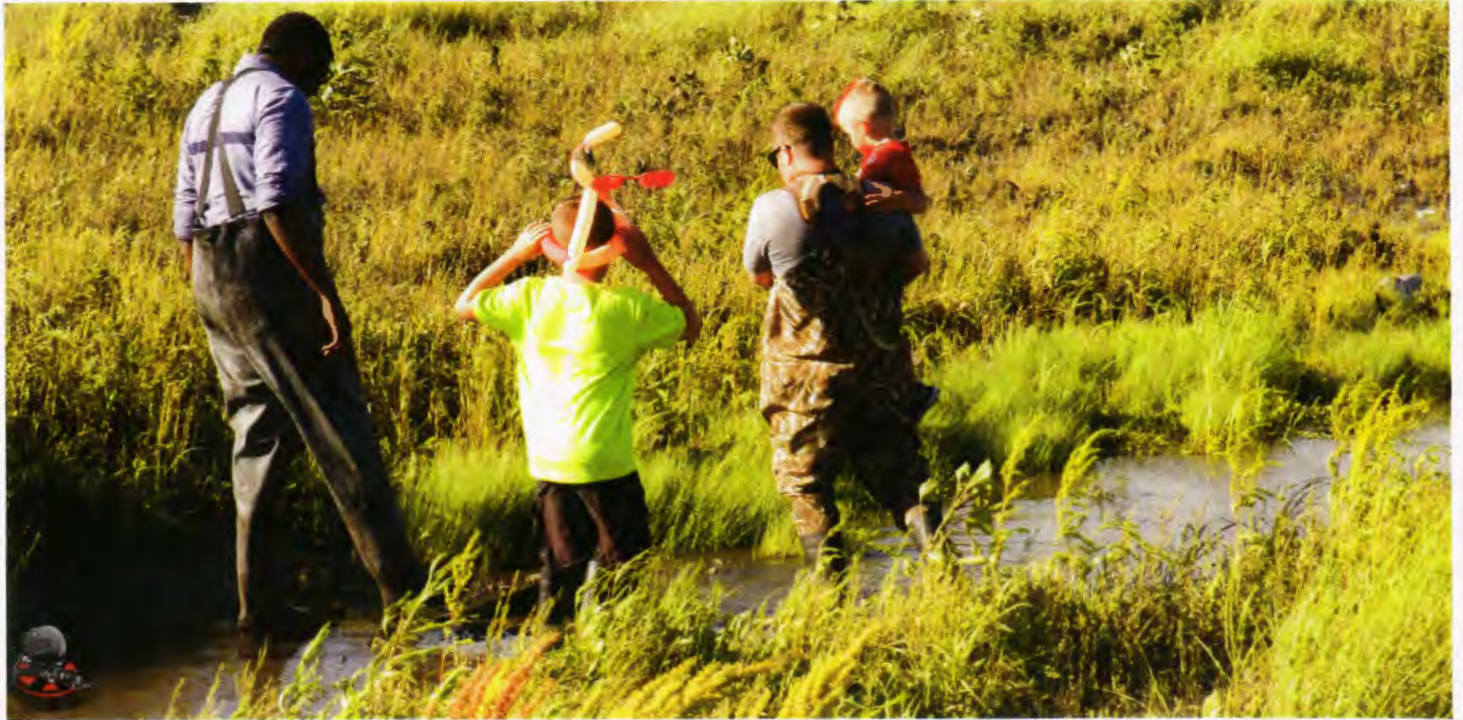
Site & vegetation restoration of area of concrete channel removal (July 2016)
