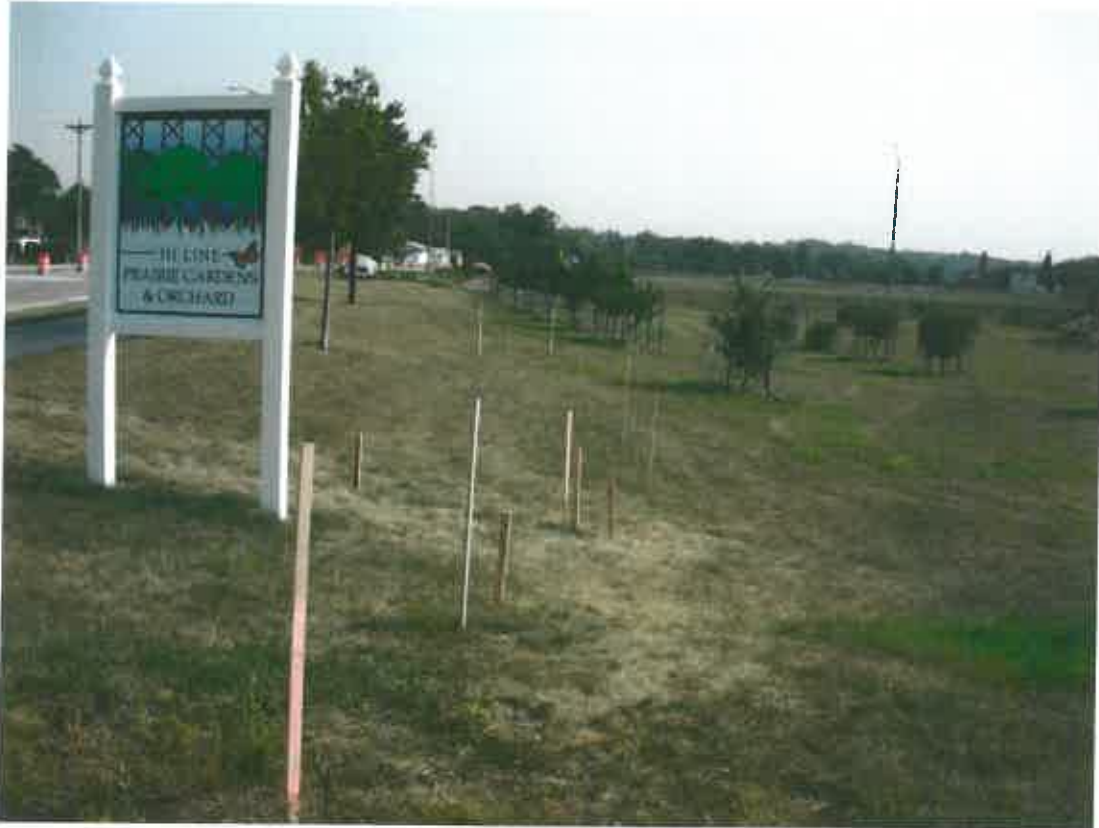
Pathways locations and elevations laid out
