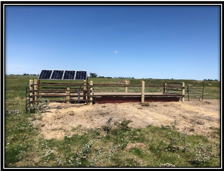
Well, Tank and Solar Pumping Station
