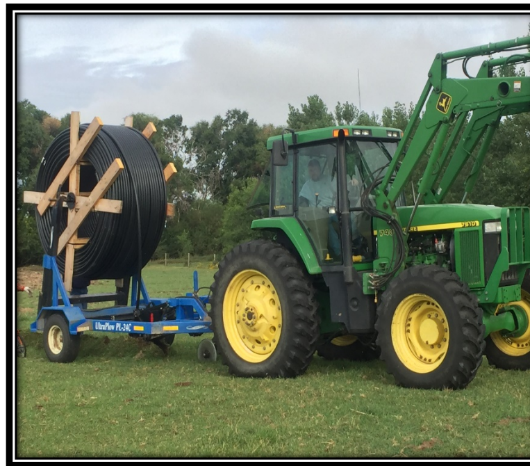
Installing shallow livestock pipeline.
