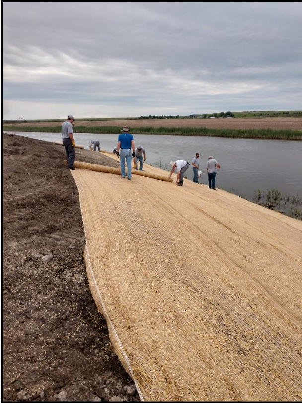
Janke James River Project – stabilization material installation
