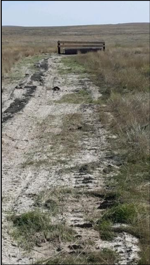
Njos Alkali Creek project – pipeline
