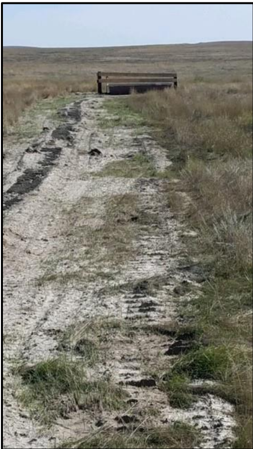
Njos Alkali Creek Project – pipeline
