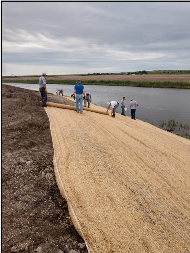
Janke James River Project – stabilization material installation
