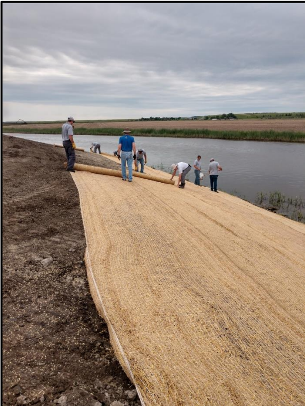
Janke James River Project – stabilization material installation
