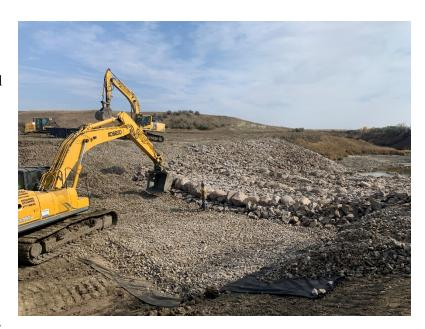
Rachel Contracting finished placing all imported material for the rock riffle structure by October 20th. The contractor removed the water control structure, topsoiled the laydown areas, finished
