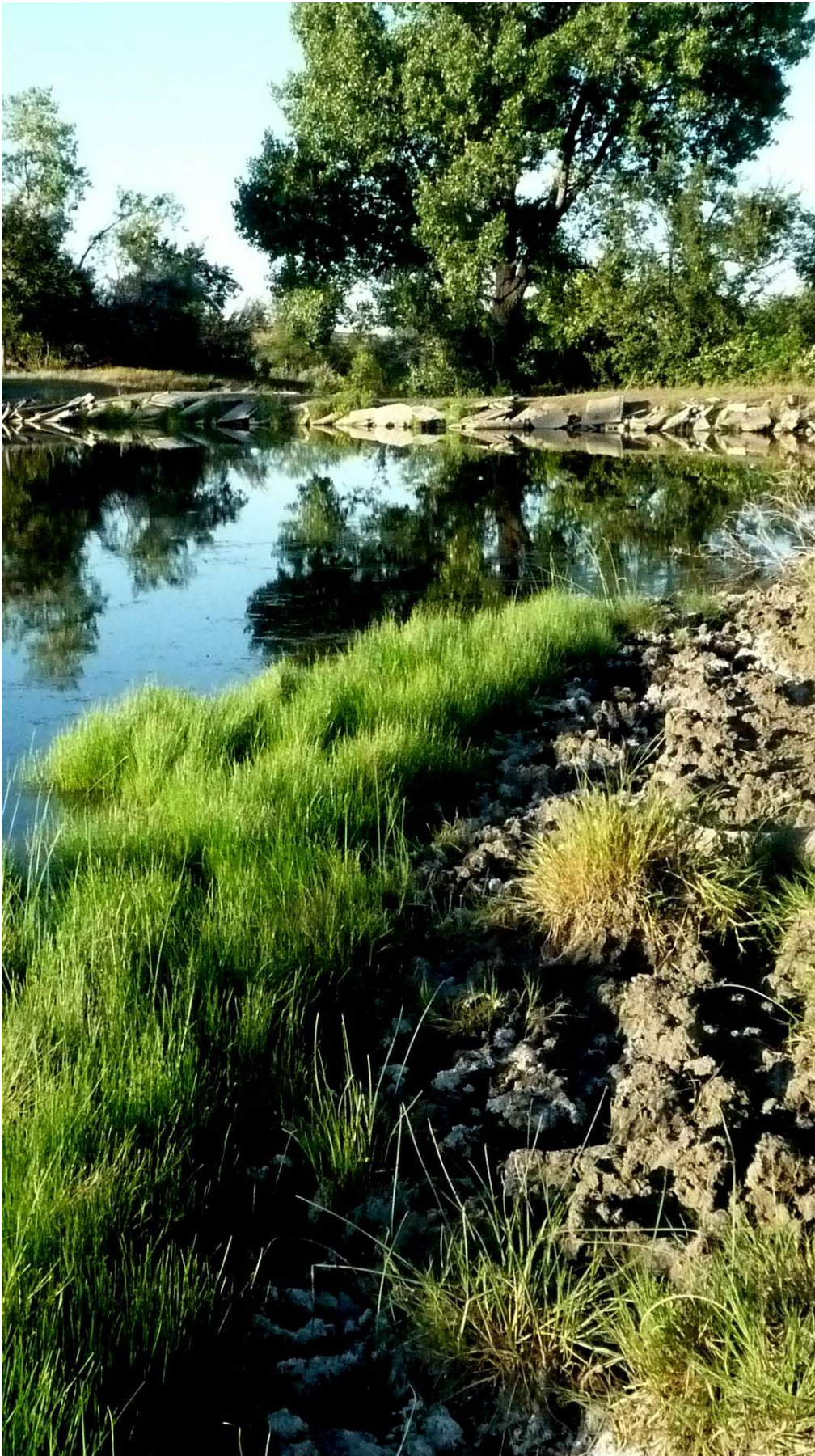
South shoreline looking east toward embankment. Note severe damage to shoreline. Landowner will bring in some topsoil to hasten recovery of shoreline areas.
