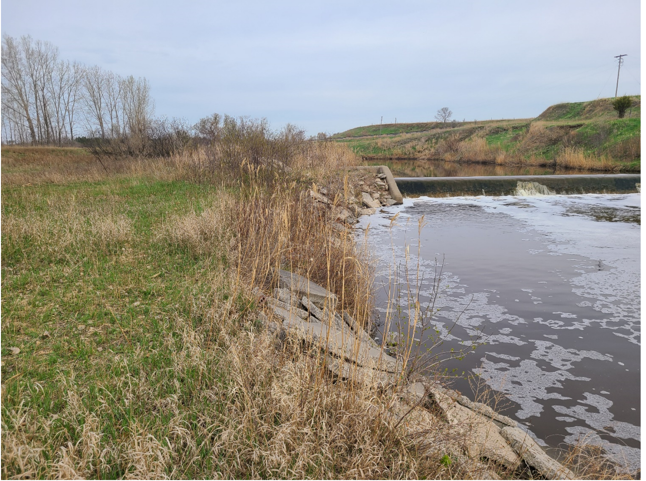
View of West Bank from Downstream of Katz Dam. The fish passage will follow the west bank around the dam.
