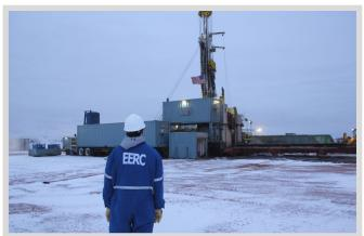
Once the permits are approved, the exploratory hole drilled in spring 2020 will be converted into the CO2 injection well. The second test site, drilled in October, will be converted into a monitoring well for the CCS project.
