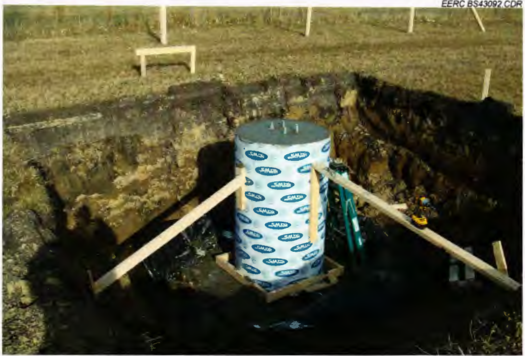
Figure 3. Winch anchor foundation.
