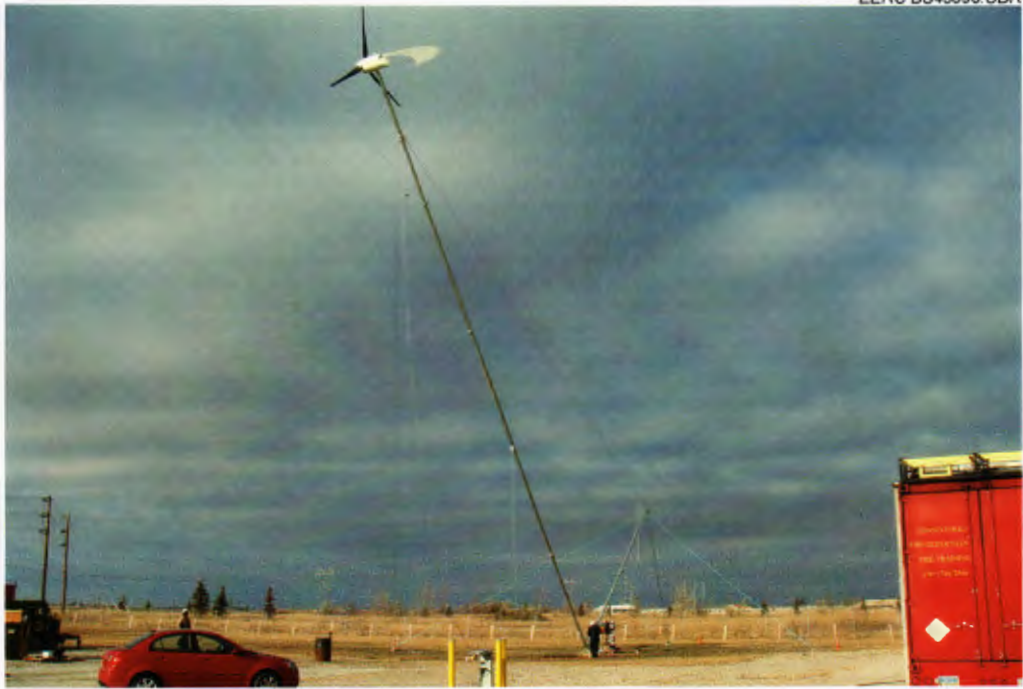
Figure 9. Fully assembled wind turbine being erected.
