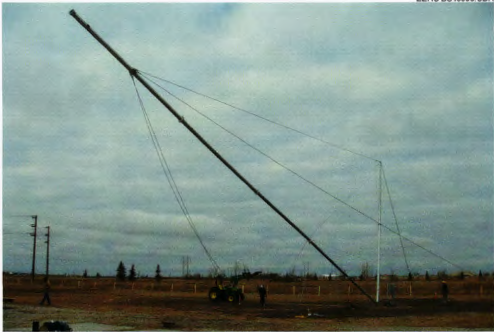
Figure 6. Tower being lifted into place (without turbine mounted).
