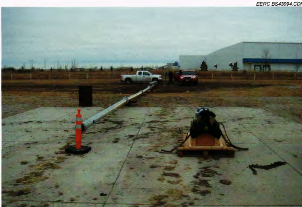
Figure 5. Tower and gin pole assembled.
