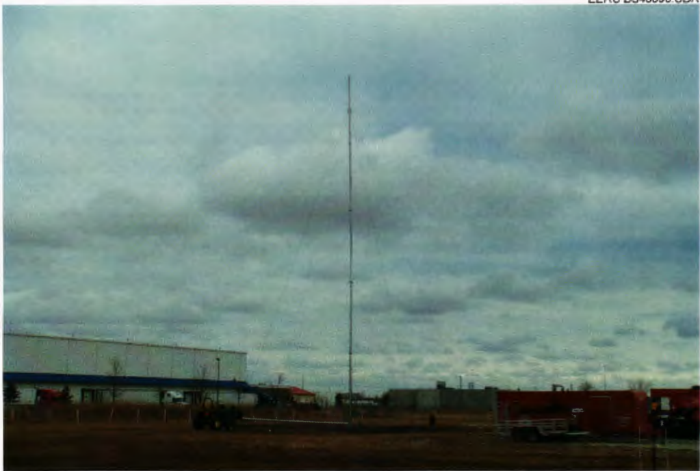
Figure 7. Tower fully erected and guy wires tensioned.
