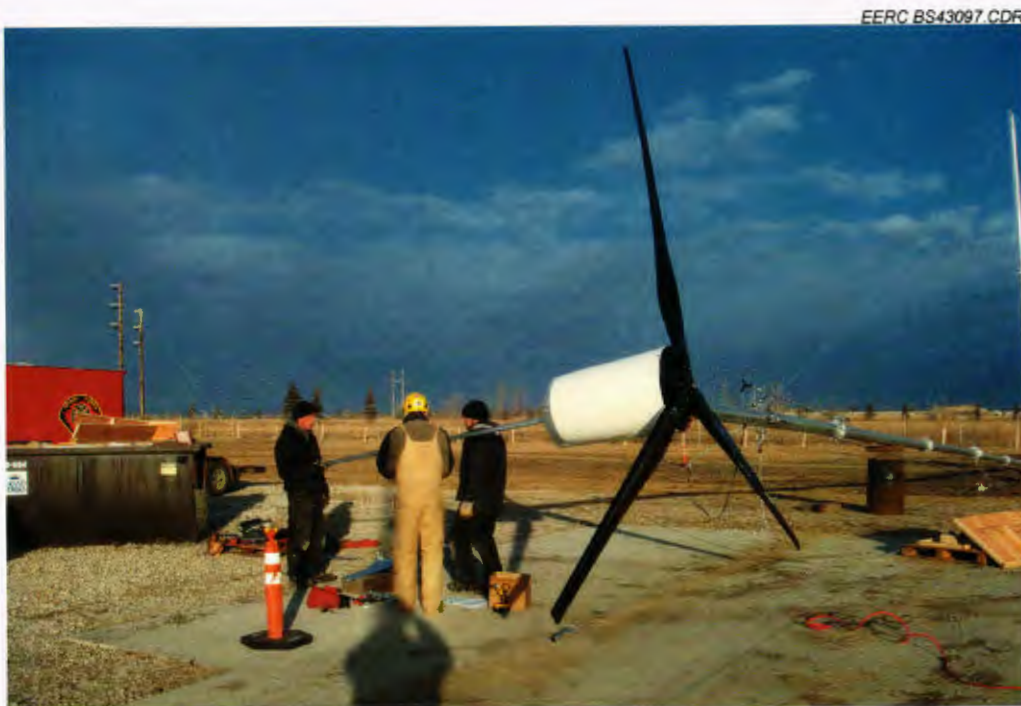
Figure 8. Mounting the turbine, blades, and tail.
