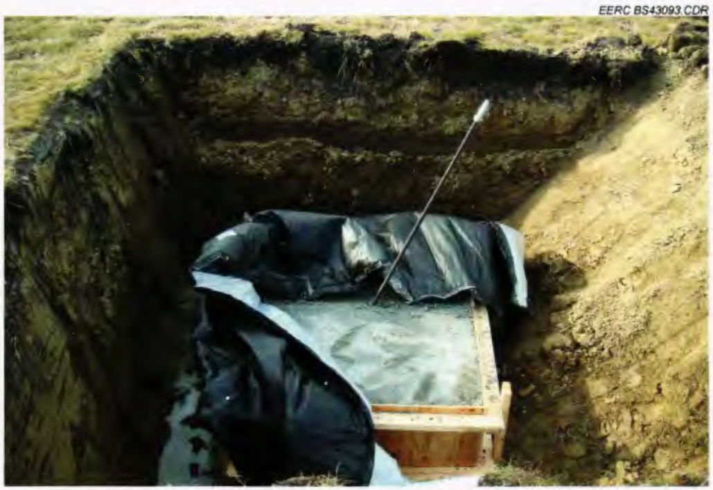
Figure 4. Guy anchor foundation.
