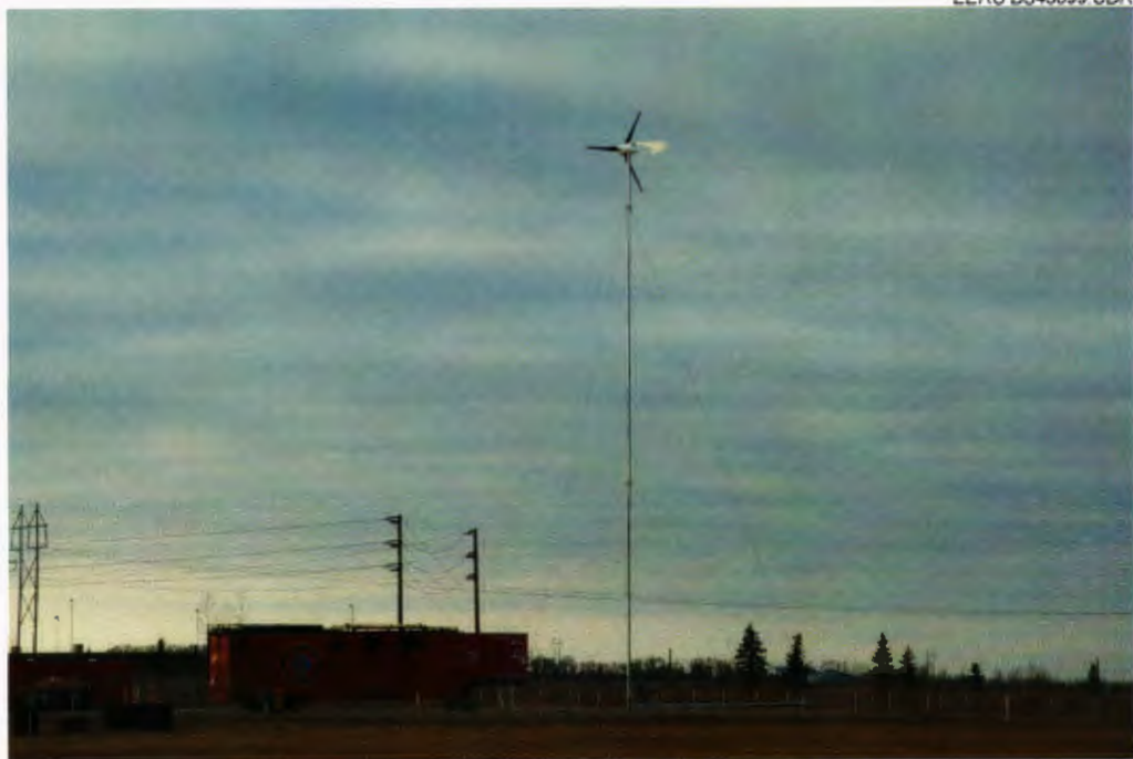
Figure 10. Wind turbine installation complete.
