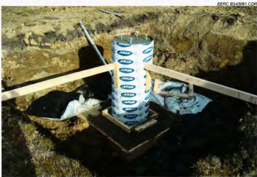
Figure 2. Tower base foundation.
