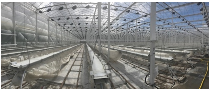
Section of Utah greenhouse being prepped for new planting
