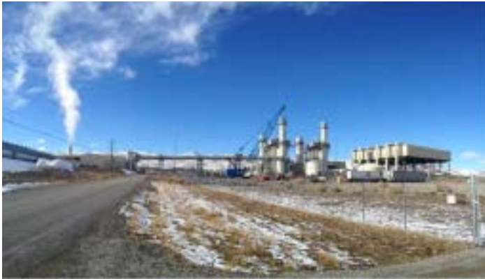
Connection between Utah greenhouse and power plant
