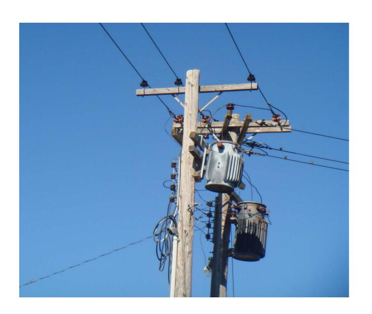
Cross arm being pulled off by transformer (arm going bad)
